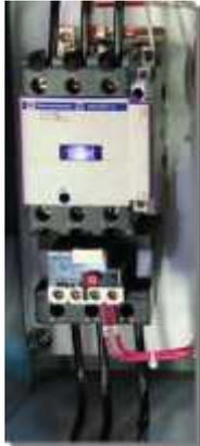
**Wash Pump trips Motor Starter Overload:** The Motor Starter Overload trips by over-ampereage. Increased amps are caused by increased load on pump motor. The most common causes are from excessive Wash Nozzle wear or excessive Throttle Bushing wear. It is possible that over-ampereage is being caused by other reasons. For help in
