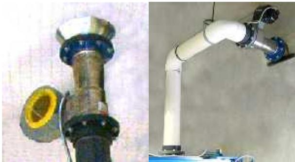
It is important that the Twist Transition be used on all vertical installations. The Twist Transition allows the blower housing motor to be in the correct position for drainage back into the steam exhaust piping and the washer.
