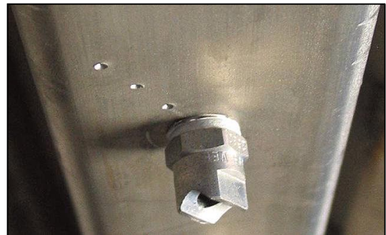
Fig. 1: Cleaning and Replacing the Power Blast Manifold Nozzles
