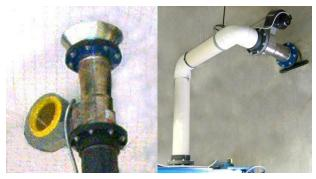
It is important that the Twist Transition be used on all vertical installations. The Twist Transition allows the blower housing motor to be in the correct position for drainage back into the steam exhaust piping and the washer. A good method to make sure of the correct orientation is to verify that the shaft of the blower motor is parallel to the floor.
